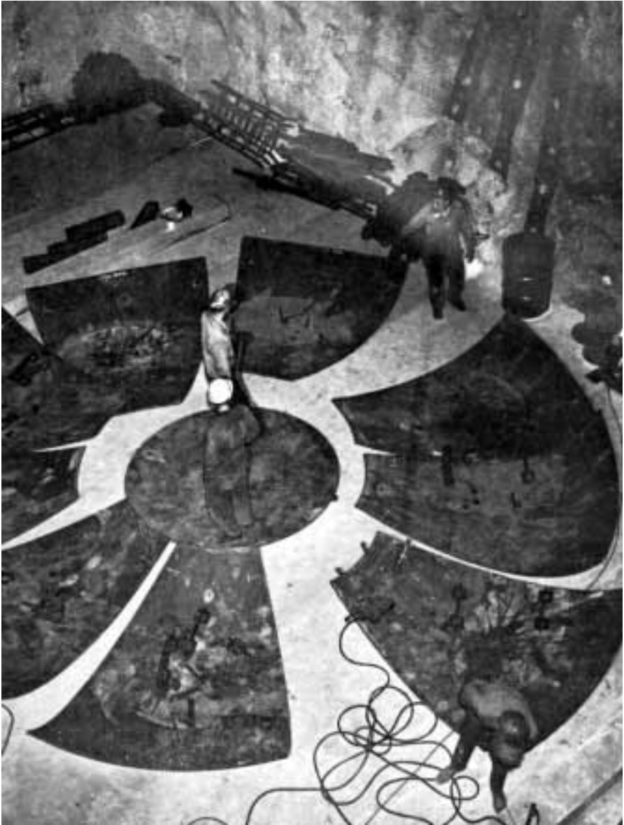
Figure 4. The pieces for one end of the tank are laid out on the floor of the big room. From Sharp Bits , June 1966.
